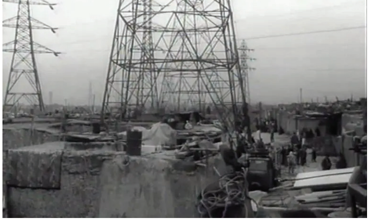
Figure 8: Documenting the slums- Marginalized families struggling for survival under hazardous pylons.
